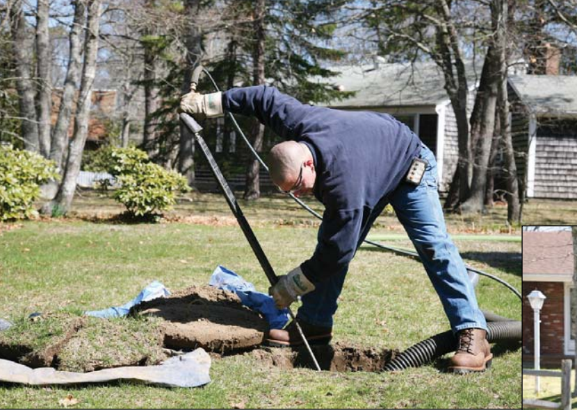
Above, technician Paul Martin jets a septic system at a residence in Hyannis, Mass. At right, Martin hooks up a hose to the Juggler truck before pumping a septic system.
